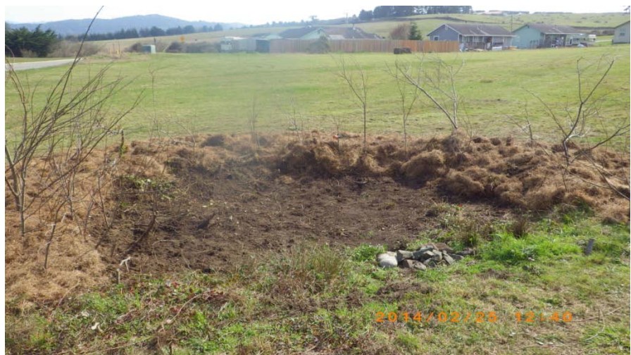
Figure 4. Stormwater retention basin on TBR treats contaminated stormwater runoff from roads/sidewalks
